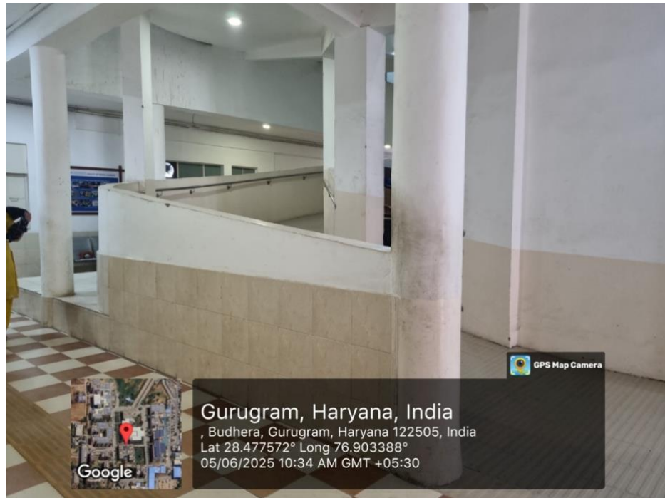
Ramp with stainless-steel handrail, view from the landing
