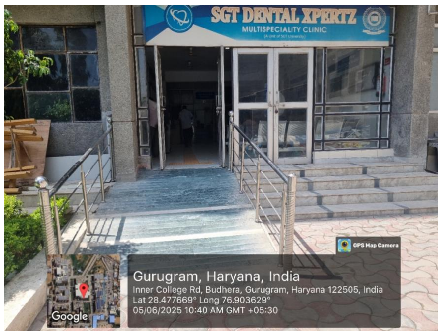
Clinic entrance with ramp and handrails (Front view)
